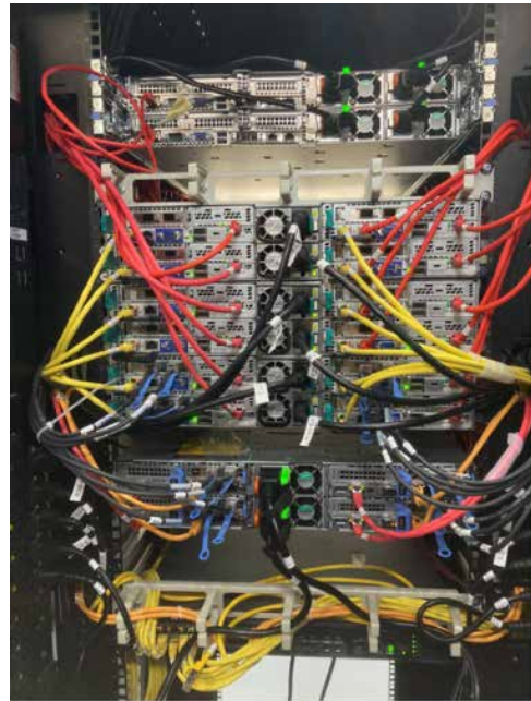
Figure 2: LAN cable colours. Black for raw data, red for LNS LAN and yellow for the control/management.
